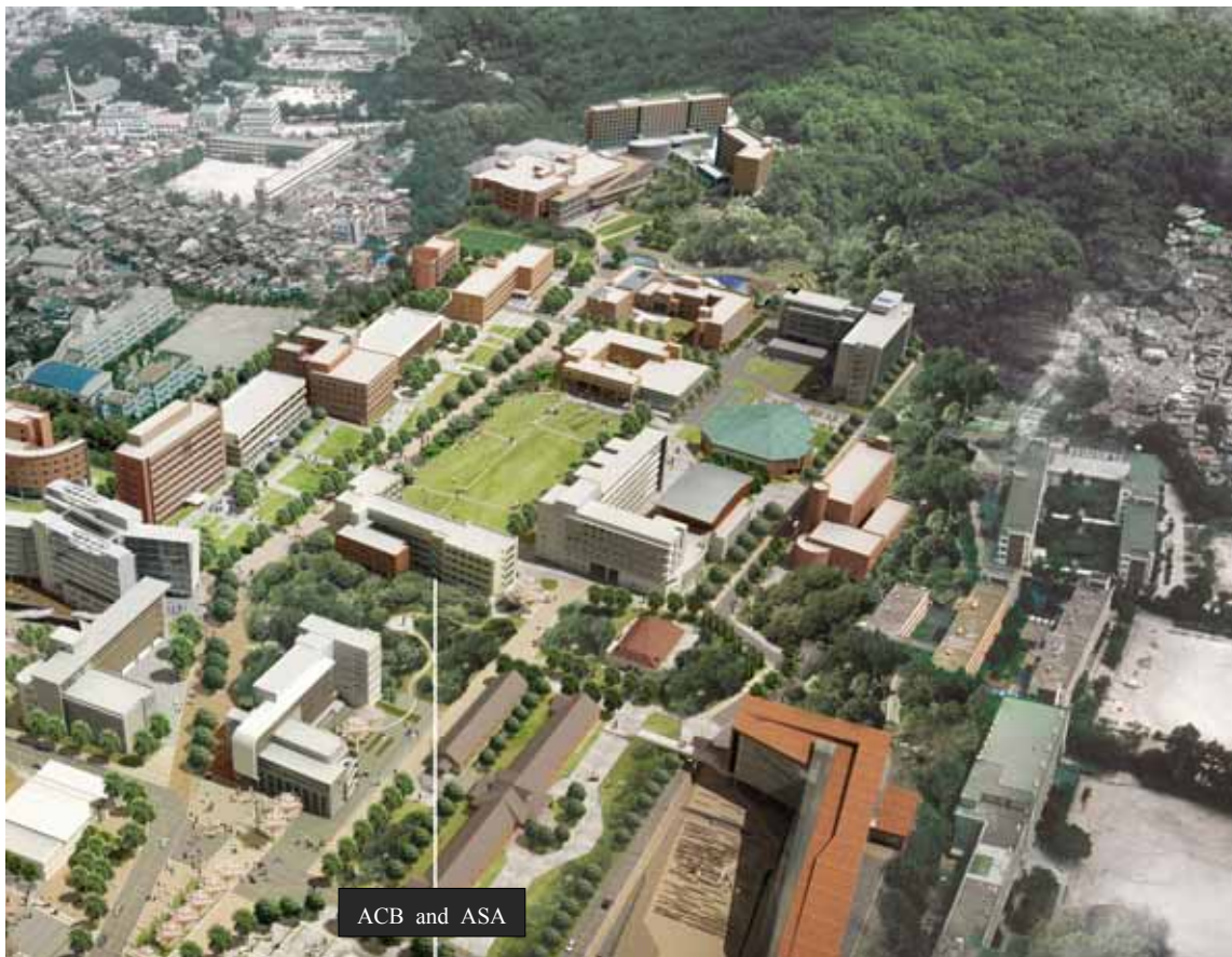
Figure 8-1_Aerial View of University of Seoul Campus, projected for 2010
